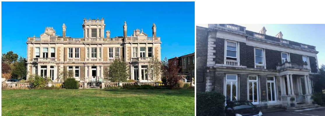
Figure 2: Photos of rear and side elevations
